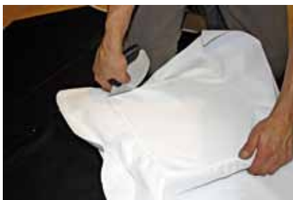
2. Clip the fabric into the profile
