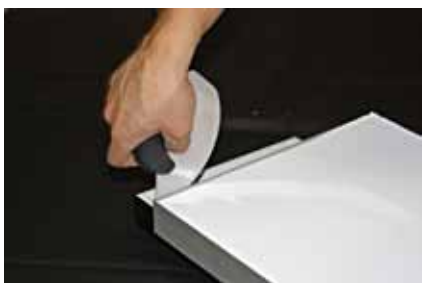
7. Tuck the margin into the profile
