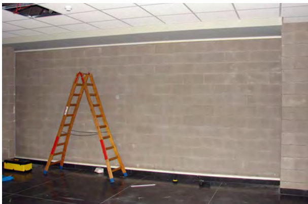
Picture of P-CC profiles fixed onto a hard surface.
