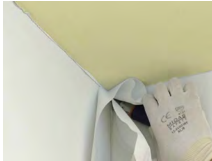
For corners, use a utility knife to remove the rest of the covering.
