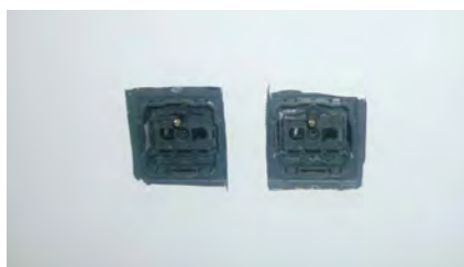
Cut into the covering.
