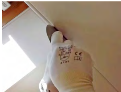
Cut into the covering.
