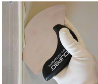
Clipping the covering into the profile.
