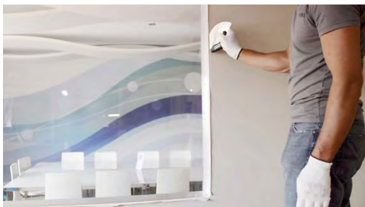
Press in the remaining excess.
