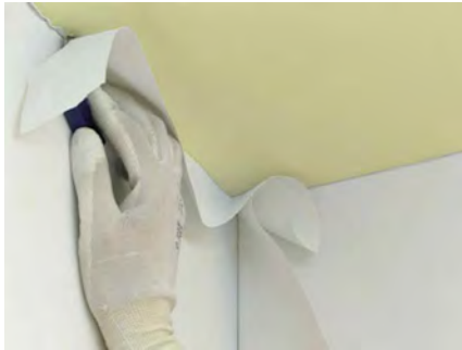
Trim the covering over the entire length using a utility knife.
