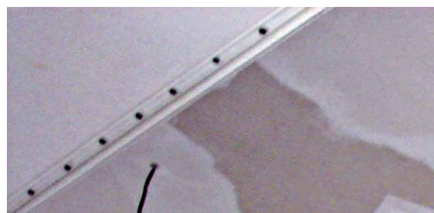
Picture of P-CC profiles fixed onto a soft surface.
